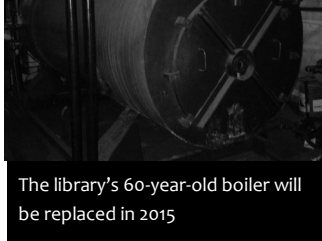
The library's 60-year-old boiler will be replaced in 2015
